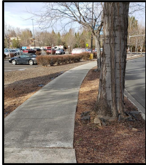
Figure 8 – The additional space available should have allowed greater space between the tree and the sidewalk.
