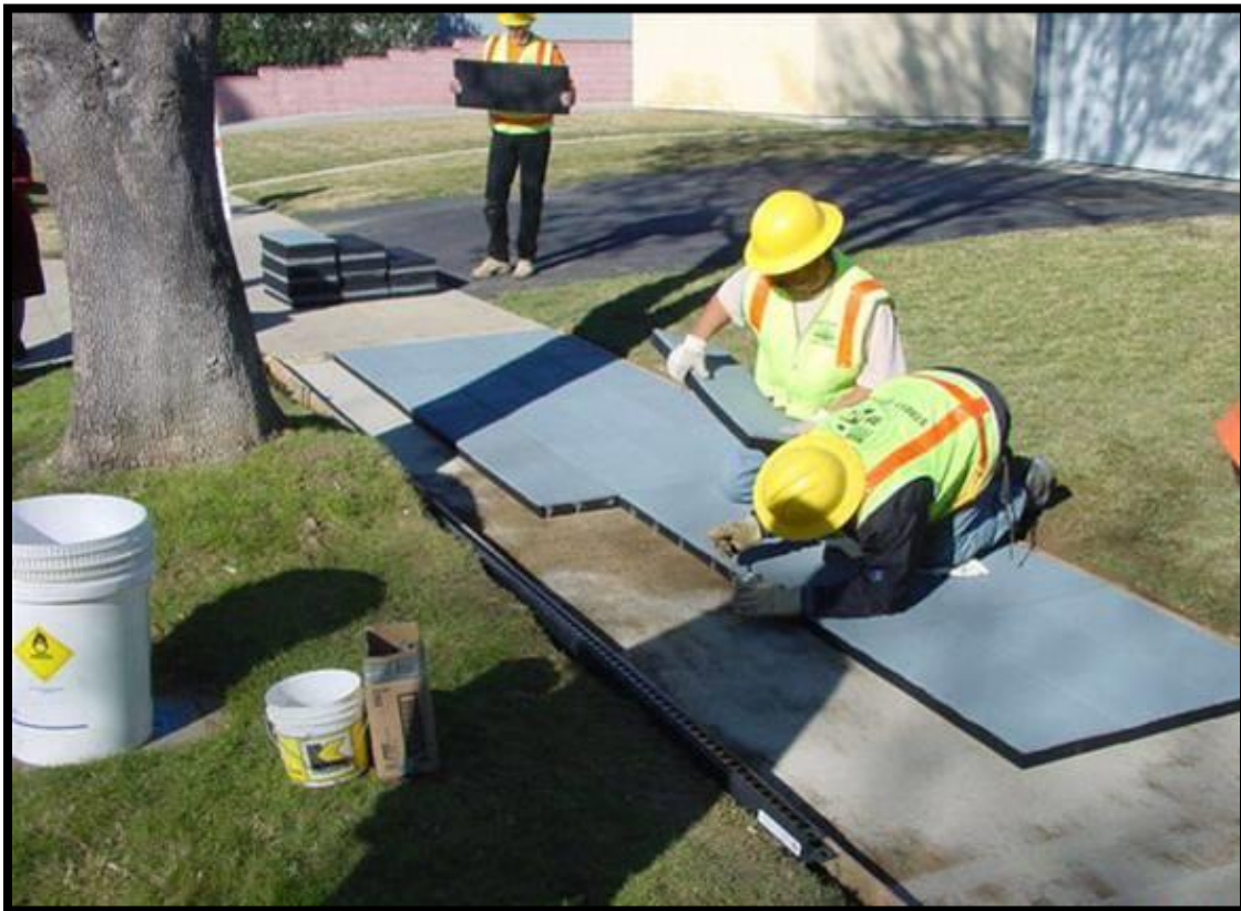
Rubber sidewalk installation.
