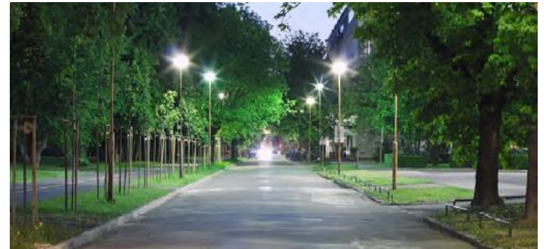
Figure 34: Lighting along a segment of roadway; image source: Marin County
