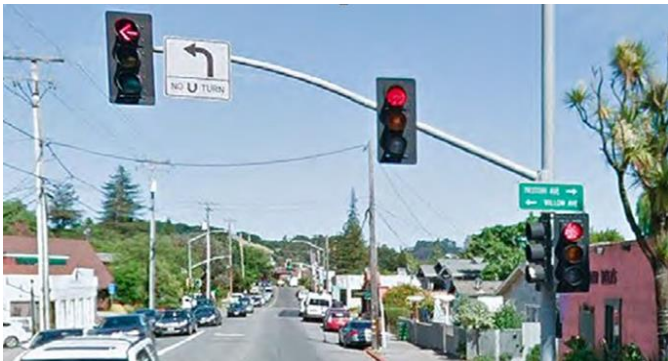
Figure 21: Protected left turn accompanied by left turn lane; image credit: Marin County
