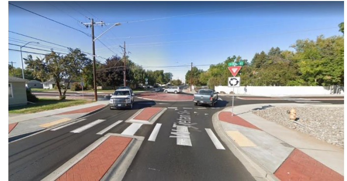
Figure 22: Mini Roundabout on 3rd Ave. and Tietan St. in Walla Walla, WA; Image Source: Google Maps
