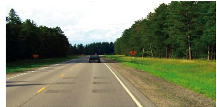
Figure 28: Transverse rumble strips (grooves) on rural road; image source: Minnesota Department of Transportation (MnDOT)
