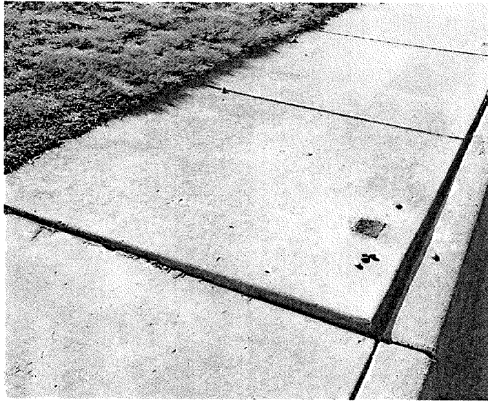
Figure 24: Curb Damage
