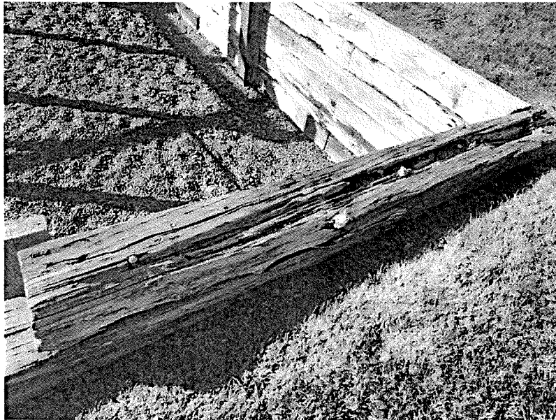
Figure 9: Retaining Wall Condition
