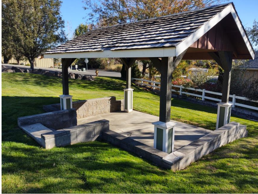
Figure 11: Shelter Concrete Pad
