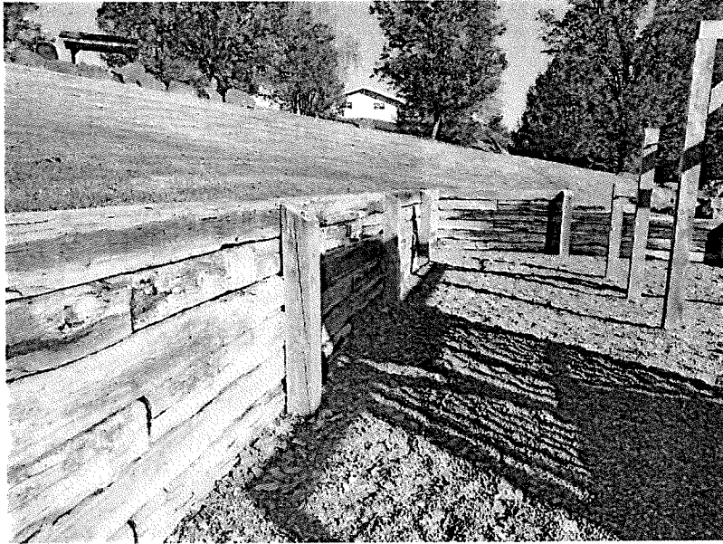
Figure 7: Park Retaining Wall
