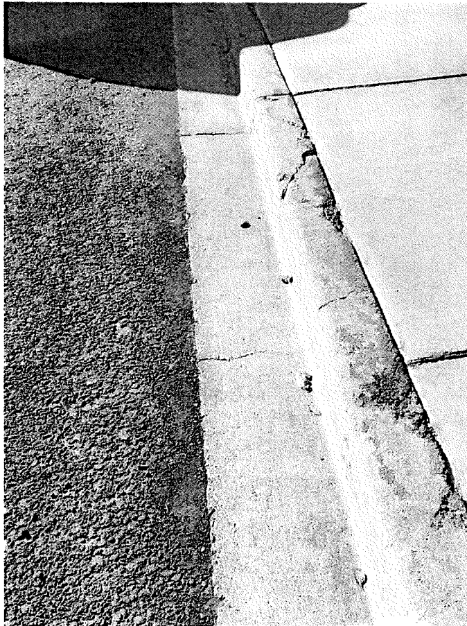
Figure 24: Curb Damage
