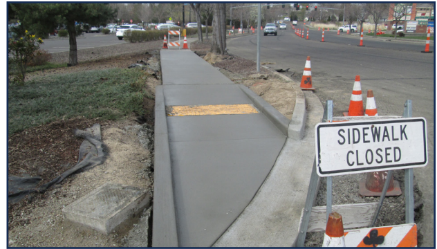
New Sidewalk on Meadowbrook Blvd, City of College Place, WA; Kate Thompson also served as the Project Manager for this project, as well as the Lamperti Street project located nearby.
