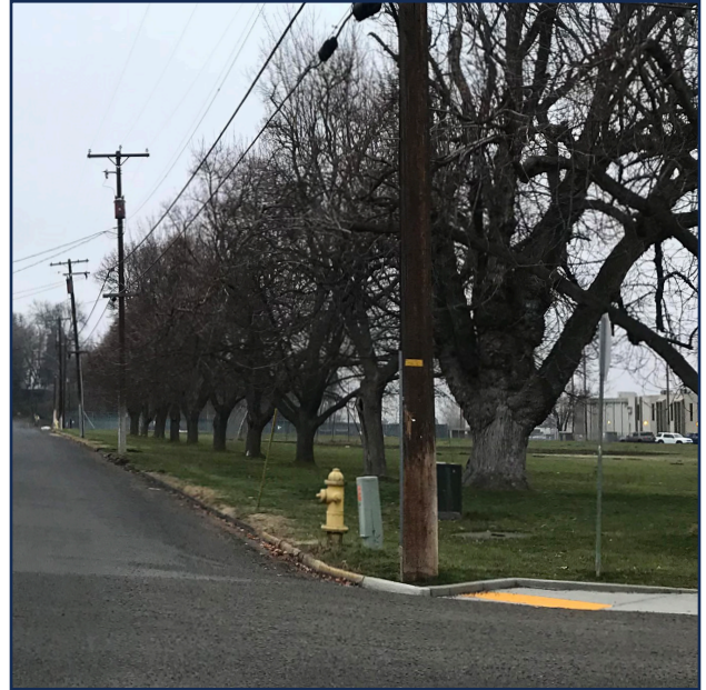
Conflicting Power Pole on the Corner of SW 6th Street and Bade Avenue, City of College Place, WA
