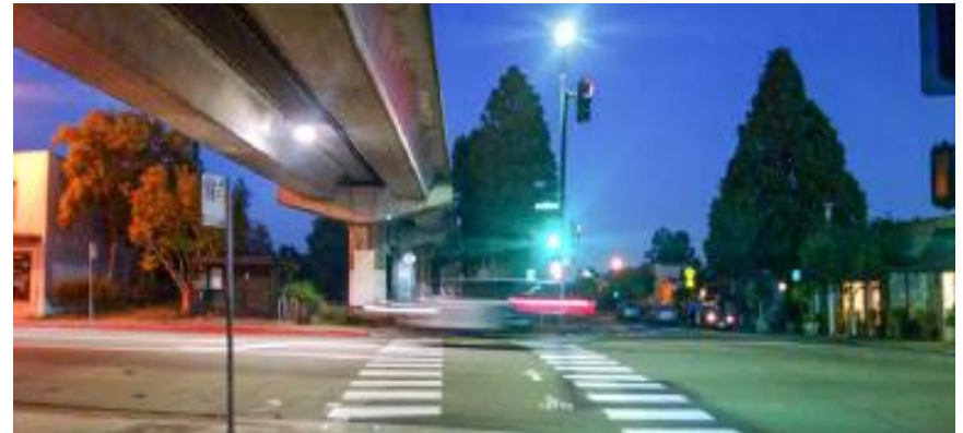
Figure 15: Lighting at intersection; image source: Marin County
