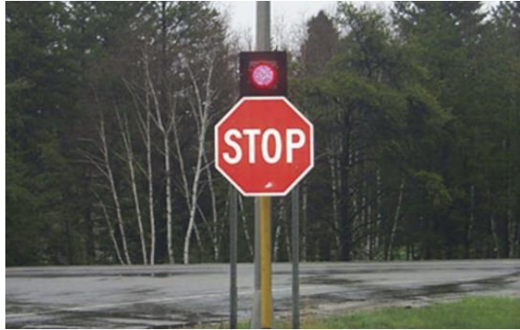
Figure 26: Flashing beacon on top of stop sign; image source: FHWA
