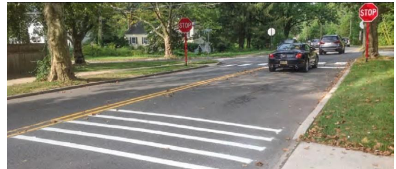
Figure 29: Transverse rumble strips on suburban road; image source: Marin County
