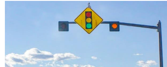
Figure 18: A flashing beacon; image source: Marin County
