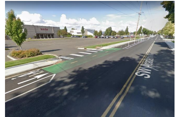
Figure 52: Pavement markings including green bike lane along 4th Ave. in College Place; image source: Google Maps
