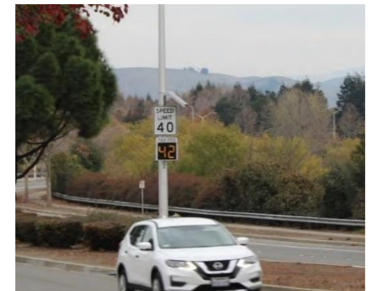
Figure 40: Dynamic speed warning sign below speed limit sign; image source: City of Fresno
