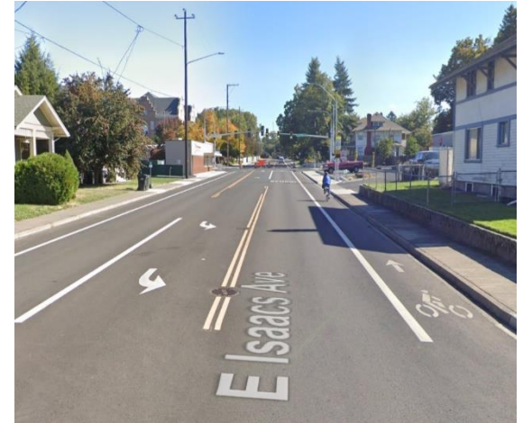
Figure 51: Bike lane along E. Isaacs Ave. in Walla Walla; image source: Google Maps
