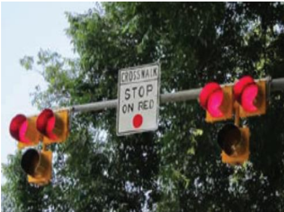
Figure 46: Pedestrian Hybrid Beacon (PHB); image source: FHWA
