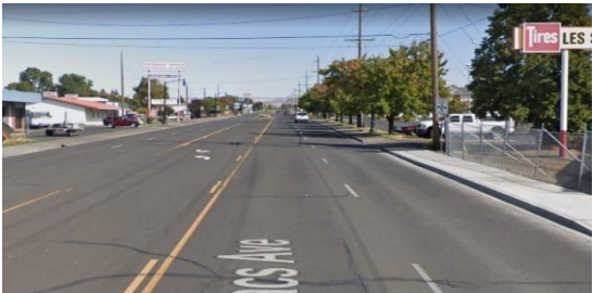
Figure 35: Two-way left turn lane in Walla Walla; image source: Google Maps
