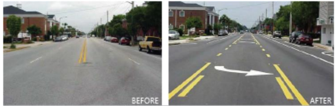
Figure 31: Before and after images of a lane conversion / road diet; image source: FHWA
