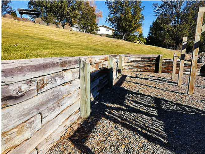
Figure 7: Park Retaining Wall
