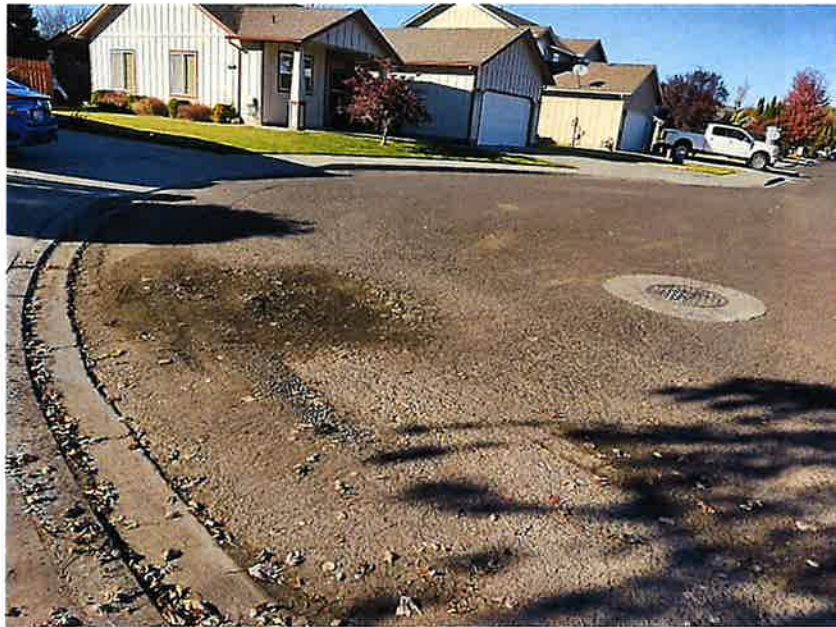
Figure 22: Pavement Condition - S.E. Newgate Court
