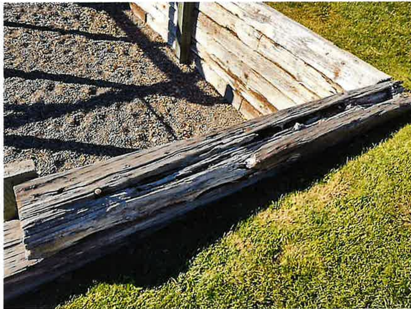
Figure 9: Retaining Wall Condition
