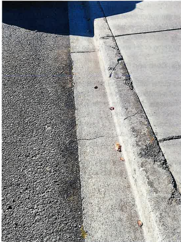
Figure 24: Curb Damage
