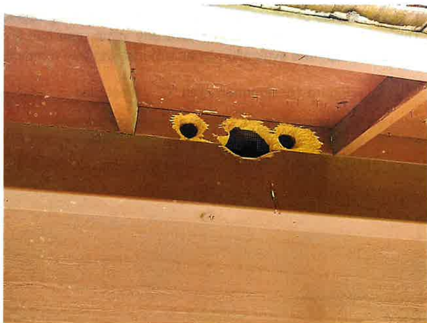
Figure 13: Pest Access - Soffit of Picnic Shelter
