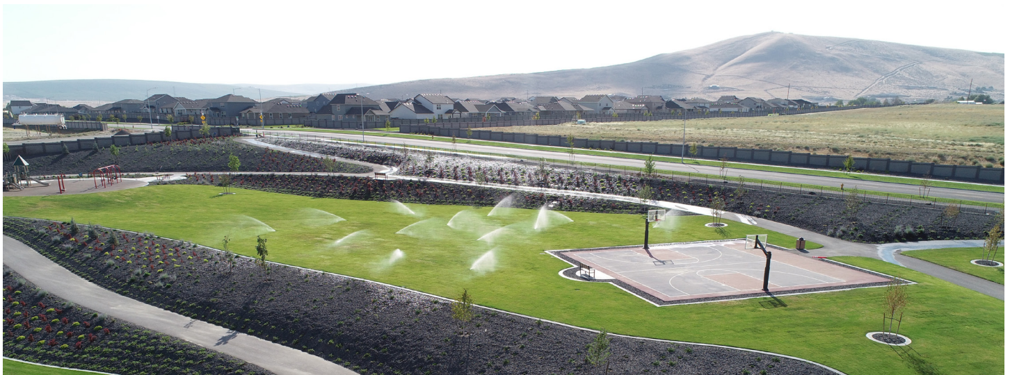
Photo 3-1. PBS designed the City of West Richland's 7-acre The Heights at Red Mountain Ranch Park within the Red Mountain Residential Subdivision. Park construction was completed in 2022.
