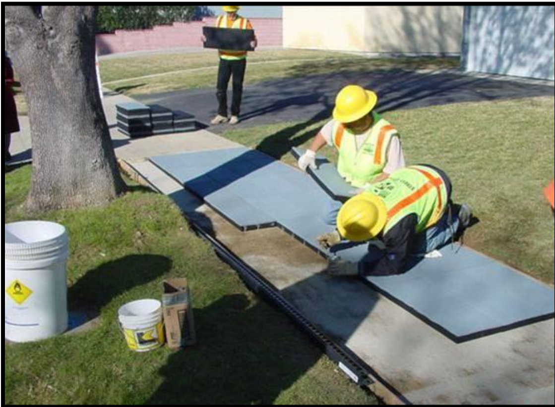
Rubber sidewalk installation.
