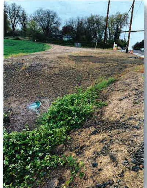
New stormwater treatment outfall structure to Stone Creek.
