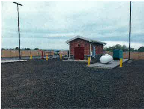
New Lift Station No. 7 site.
