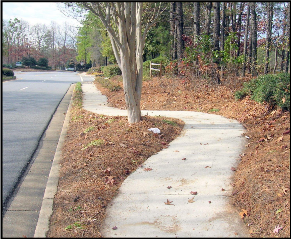
Figure 9 - Re-routing sidewalks around a large tree is a successful option.
