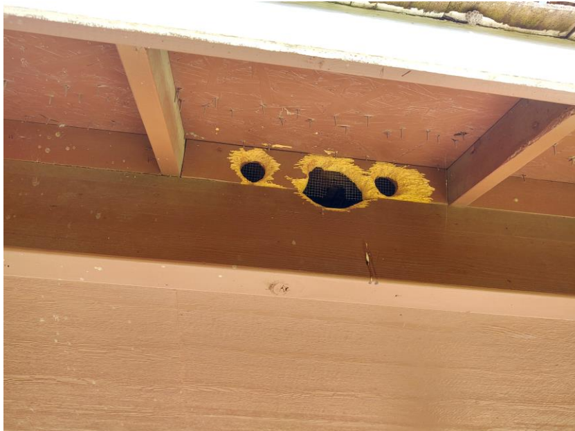
Figure 13: Pest Access - Soffit of Picnic Shelter
