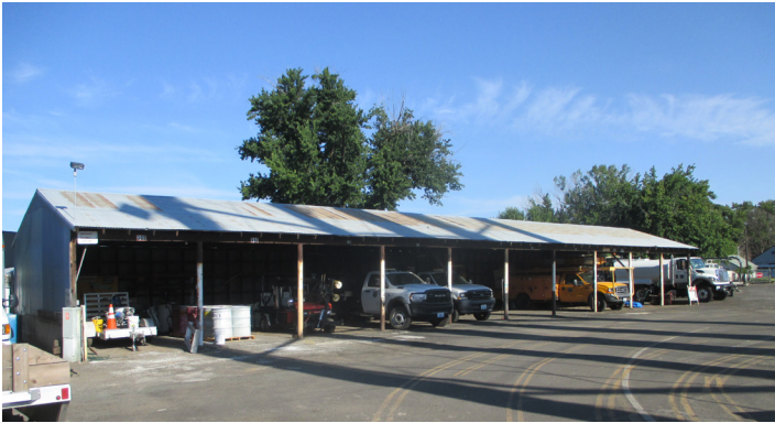
College Place Public Works Department Vehicle Storage
