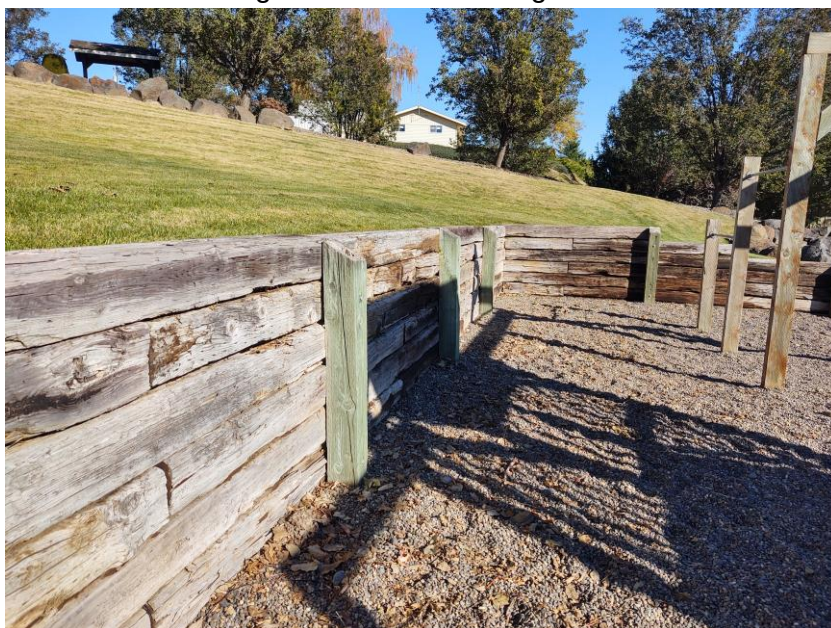
Figure 7: Park Retaining Wall
