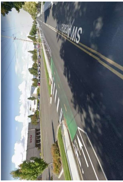
Figure 52: Pavement markings including green bike lane along 4thg Ave. in College Place; image source: Google Maps
