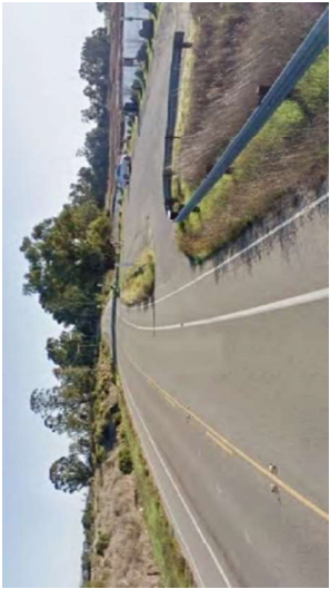
Figure 32: Clear recovery zone; image source: Marin County
