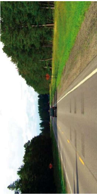
Figure 28: Transverse rumble strips (grooves) on rural road; image source: Minnesota Department of Transportation (MnDOT)
