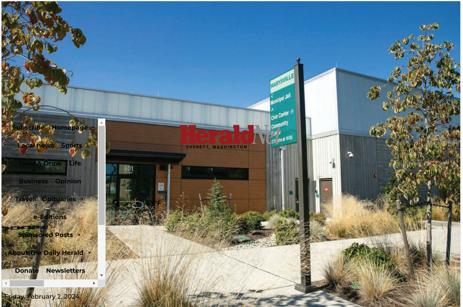
The Marysville Municipal Jail is pictured Thursday, Sept. 14, 2023, in Marysville, Washington. (Ryan Berry / The Herald)
