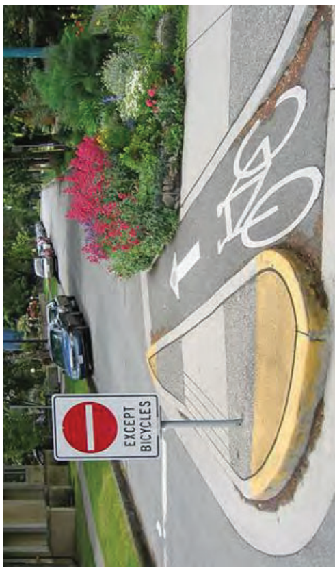
Bicycle connection through a channelization island with a do not enter except bicycles sign.
