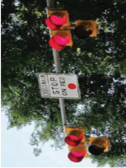
Figure 46: Pedestrian Hybrid Beacon (PHB); image source: FHWA
