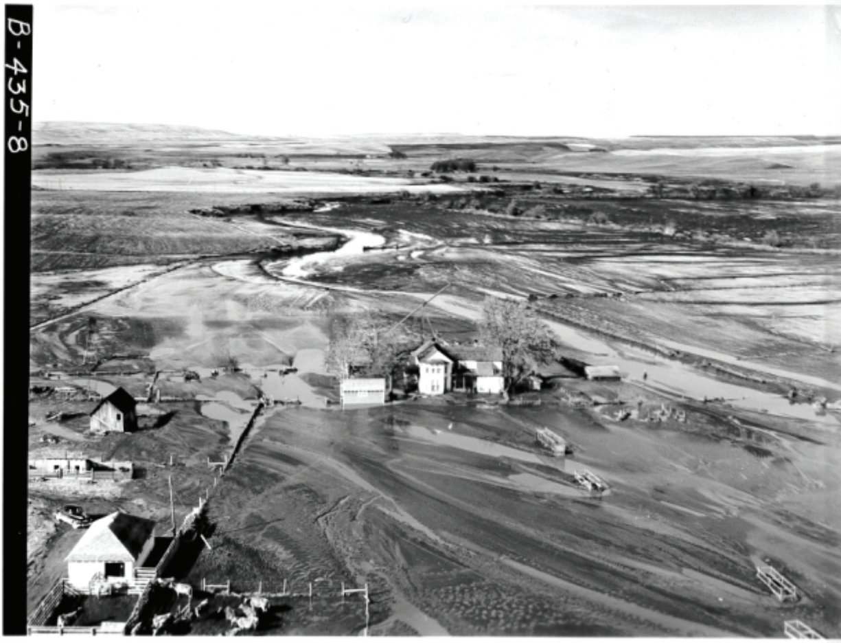
This is a USDA SCS flooding picture.
