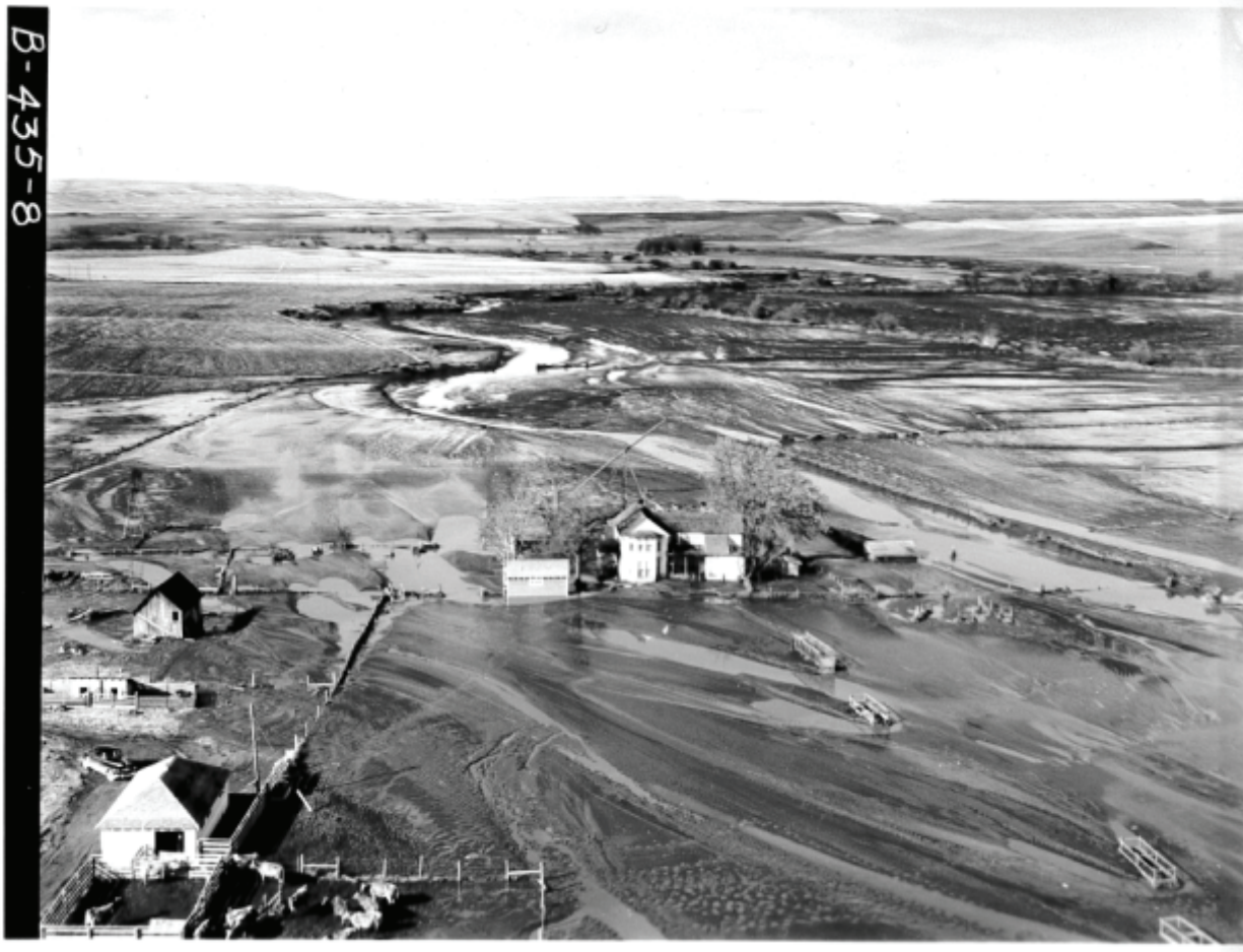
This is a USDA SCS flooding picture.
