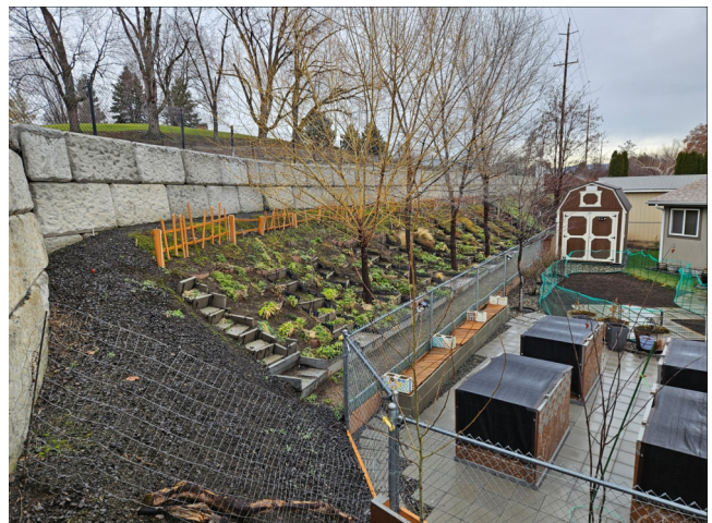
Figure 4 - VIEW FROM BELOW - LOOKING UP TO THE CURB
