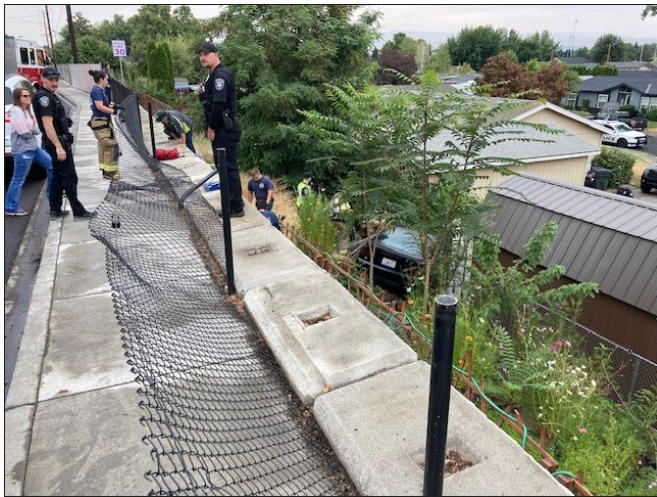
Figure 1 - VEHICLE TRAVELED THROUGH FENCE INTO PROPERTY BELOW
