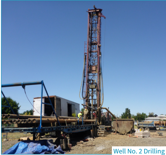
Well No. 2 Drilling
