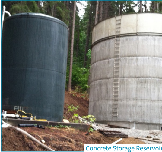
Concrete Storage Reservoir
