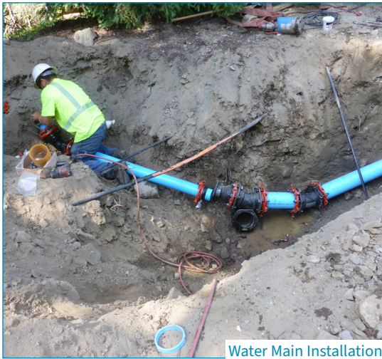
Water Main Installation
