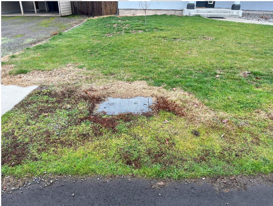
Figure 13. View of electrical box near the western edge of Damon Avenue from Photo Point #7 (Aspect: West)
