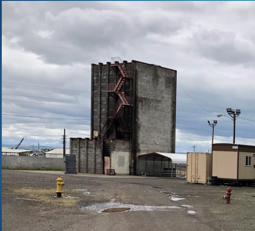
70's DRILL TOWER
