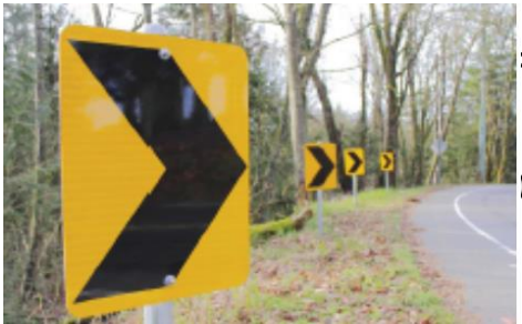
Figure 36: Chevron signs along a curve; image source: FHWA
