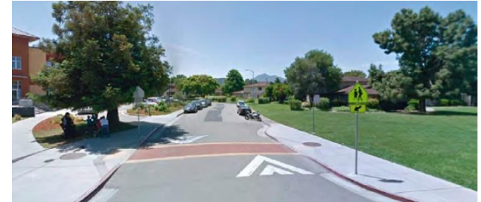
Figure 49: Raised crosswalk featuring markings and colored paving material; image source: Marin County
