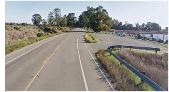
Figure 32: Clear recovery zone; image source: Marin County
