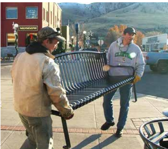
New benches being installed in downtown Chelan.
