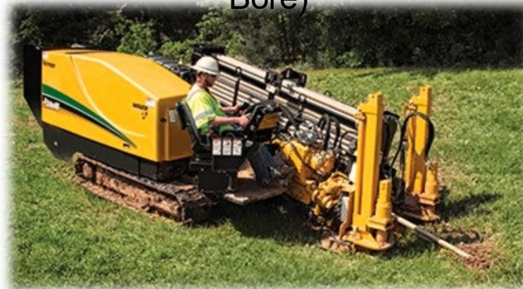
Buried Cable Placement (Directional Bore)
