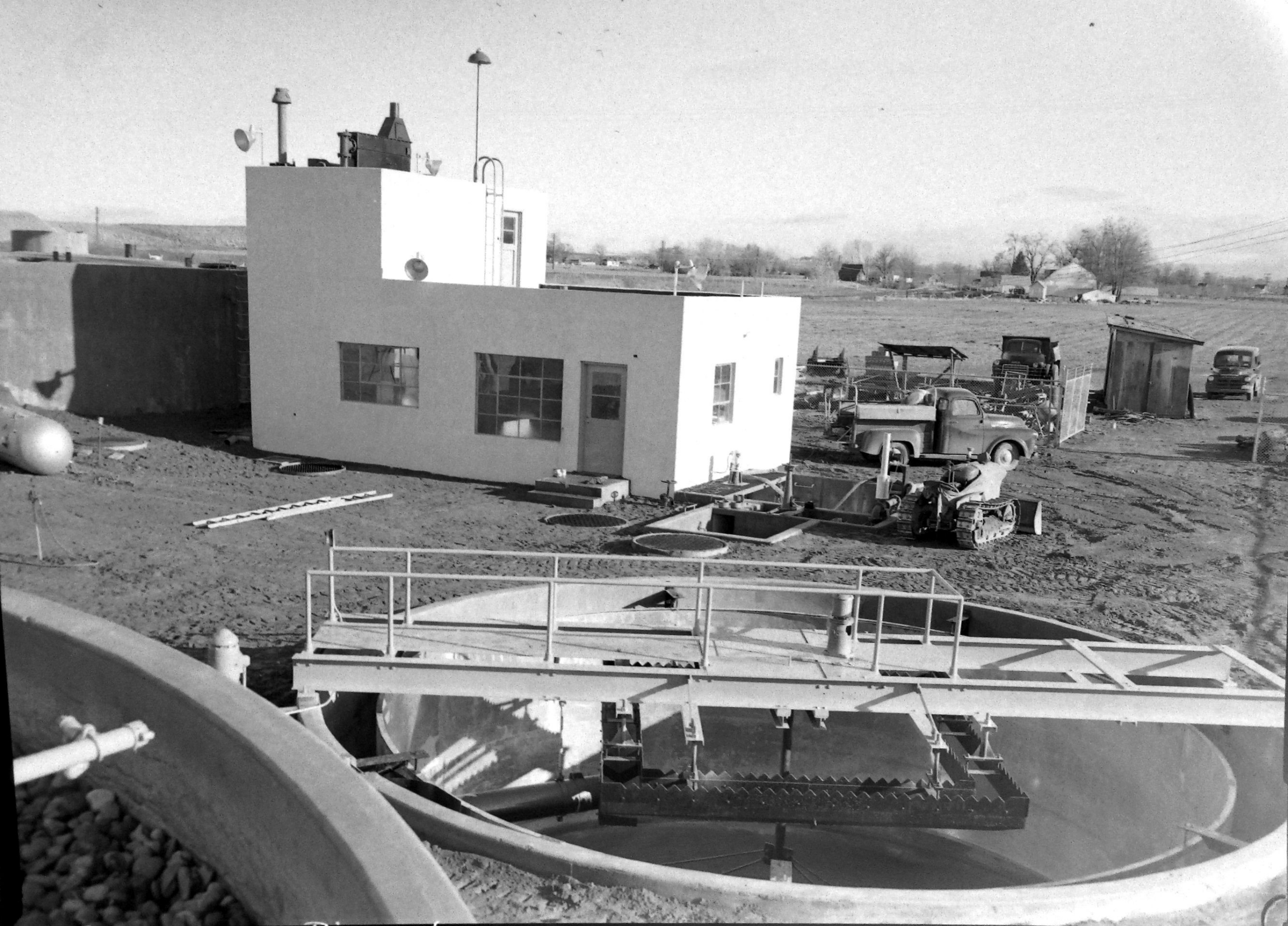
C. Place Sewer Disposal
