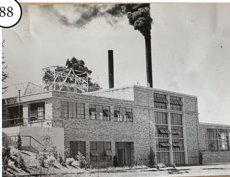
Power House, Built around 1947
