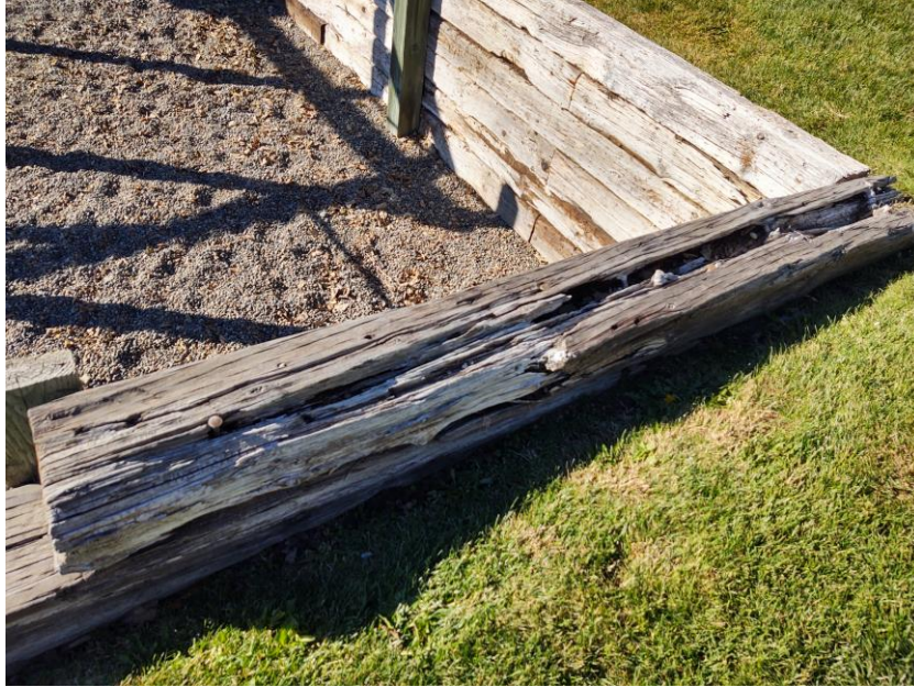
Figure 9: Retaining Wall Condition
