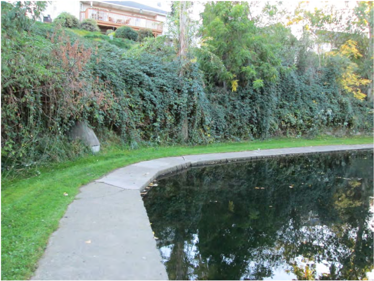
Photo 5. Stormwater inlet pipe to the fishing pond.
