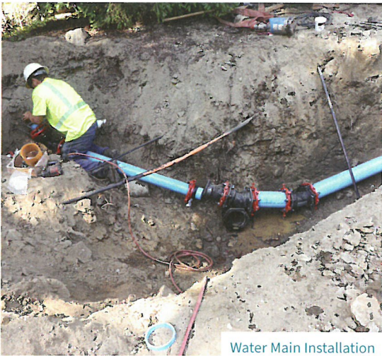
Water Main Installation
