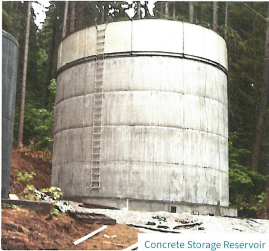
Concrete Storage Reservoir
