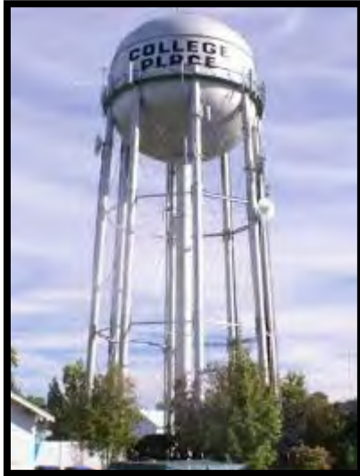
Photo 2 College Place Water Tower
