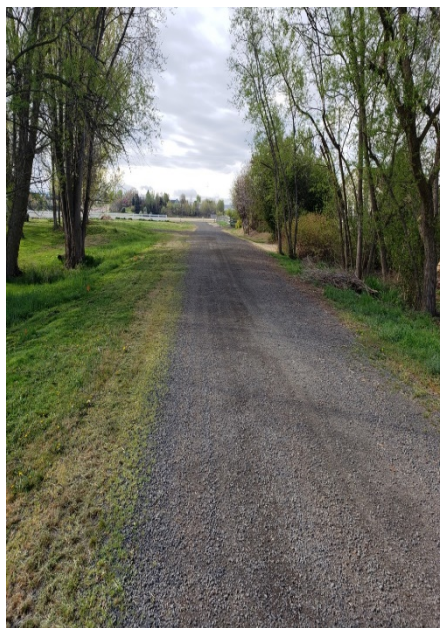
Photo 8. Western Project Corridor (facing south)
