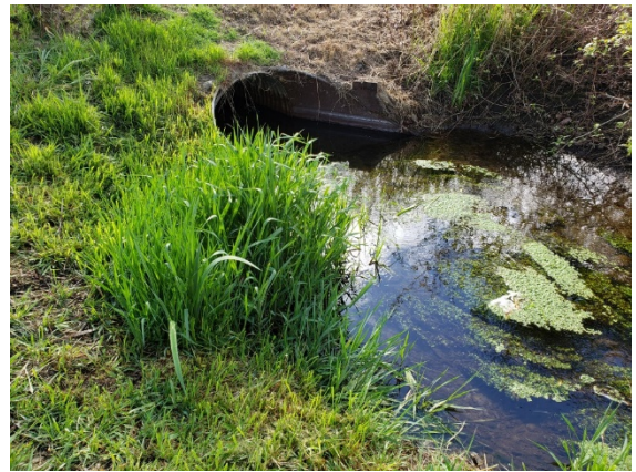
Photo 10. Existing Culvert (Upstream side)
