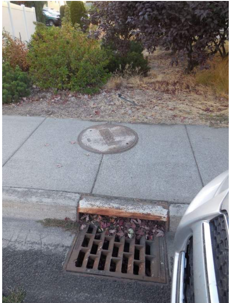
Photograph 3-1. Outfall #37 - Catch Basin Inlet - Looking West Toward Thompson Creek
