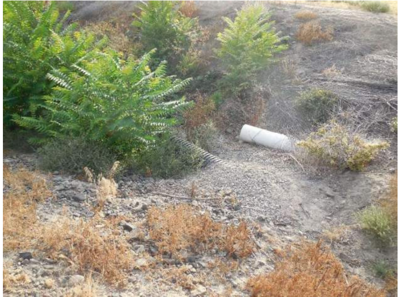
Photograph 2-12. Wetland Outfall - Two Outfall Pipes
