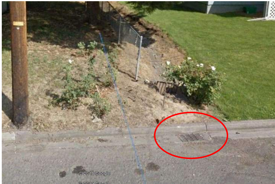
Photograph 3-3. Outfall STRUCT #406 – Catch basin into Thompson Creek (Google Earth)
