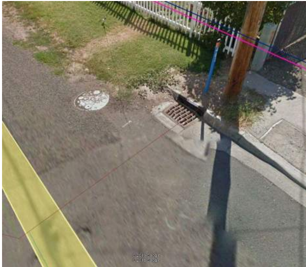
Photograph 4-1. Outfall at Lambert Avenue – north of Spitzenburg Street (Google Earth)
