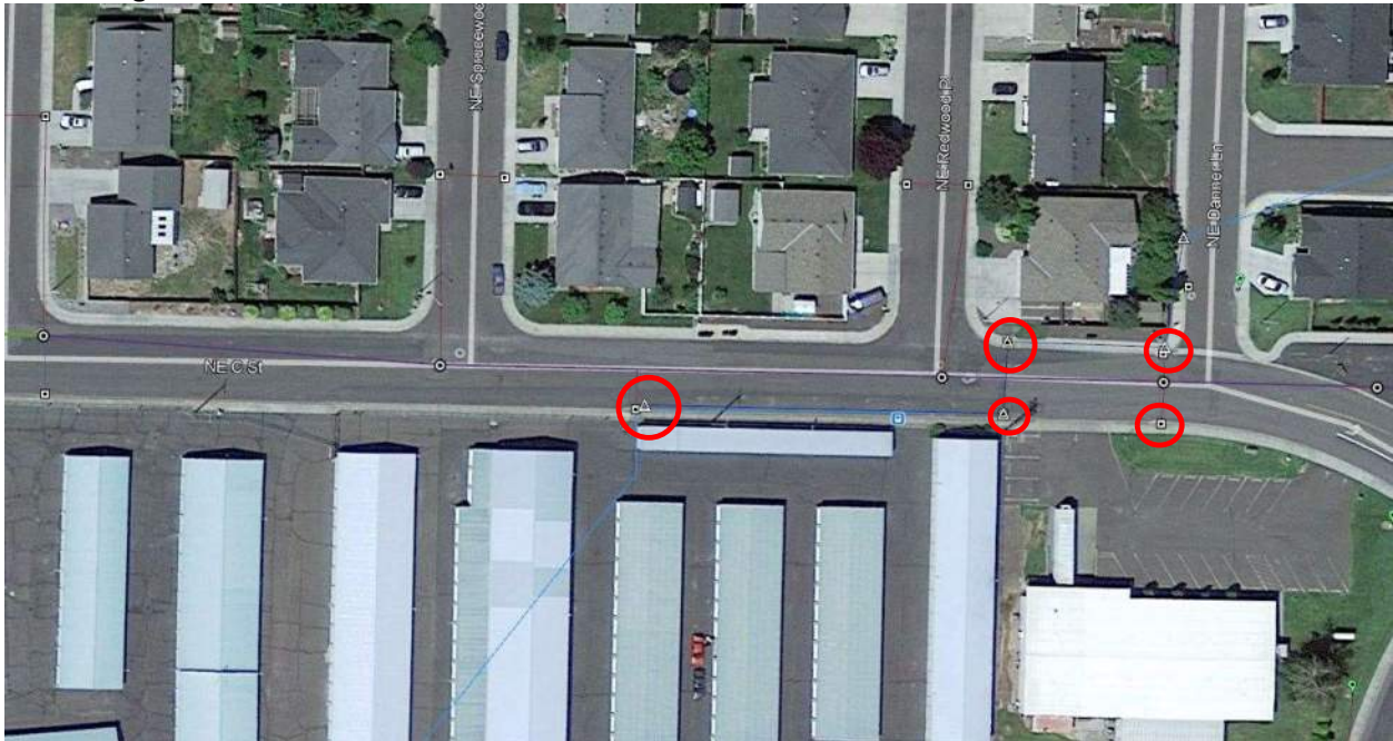
Photograph 4-3. Outfalls #50, 51, 52, 53, 54 (Google Earth)
