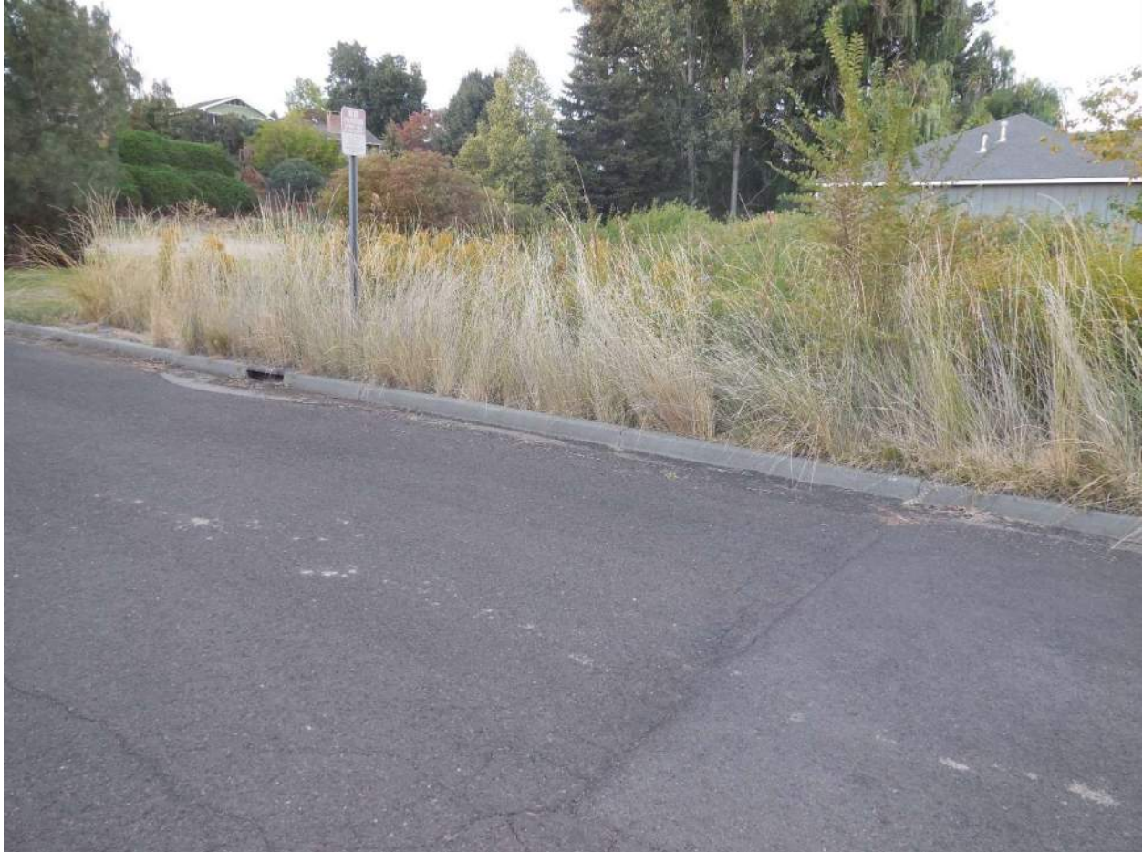
Photograph 2-17. Outfall #2 - Catch Basin with Outfall to Stone Creek Downstream
