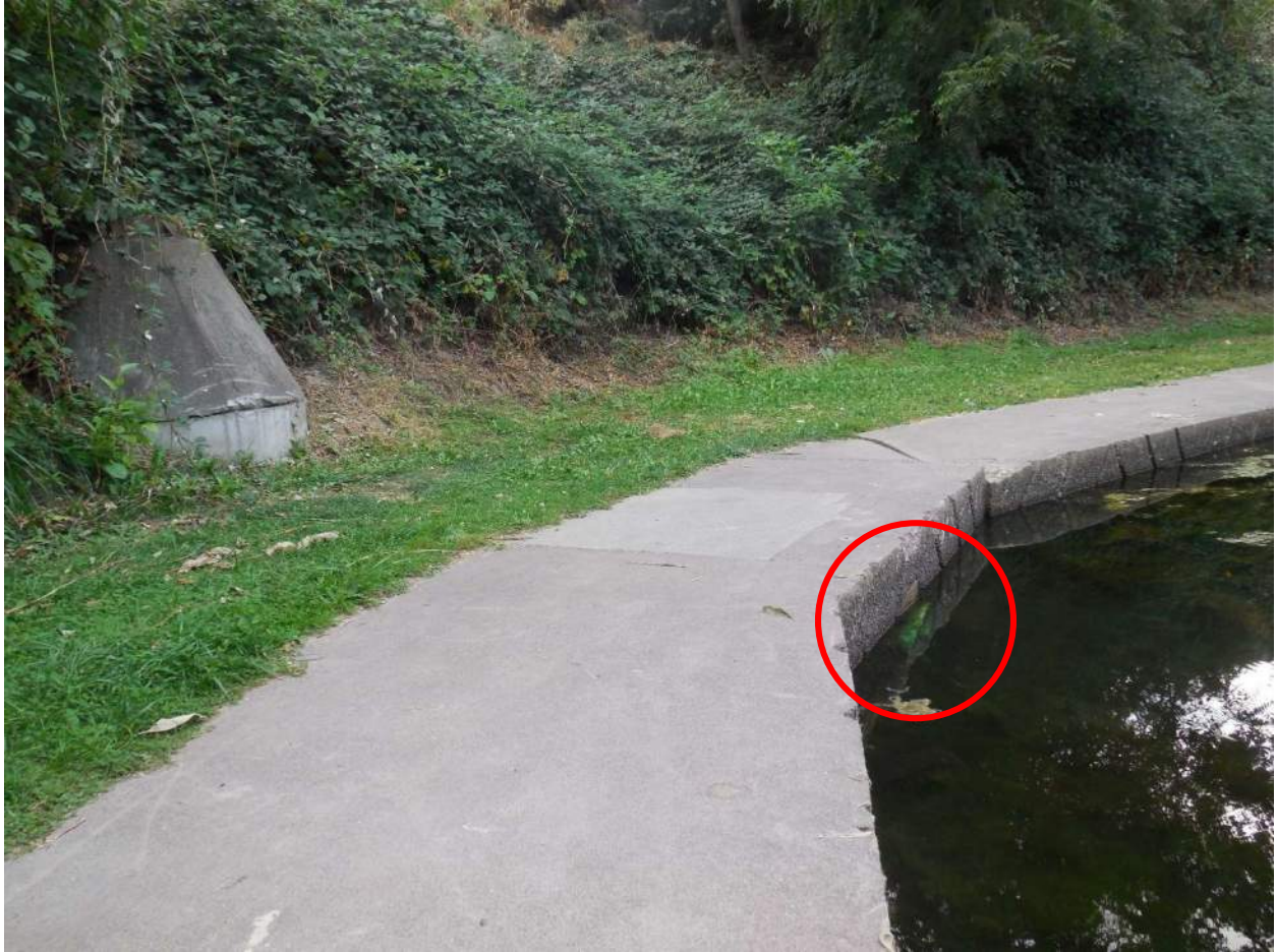
Photograph 1-16. Outfall 80 - Pond View
