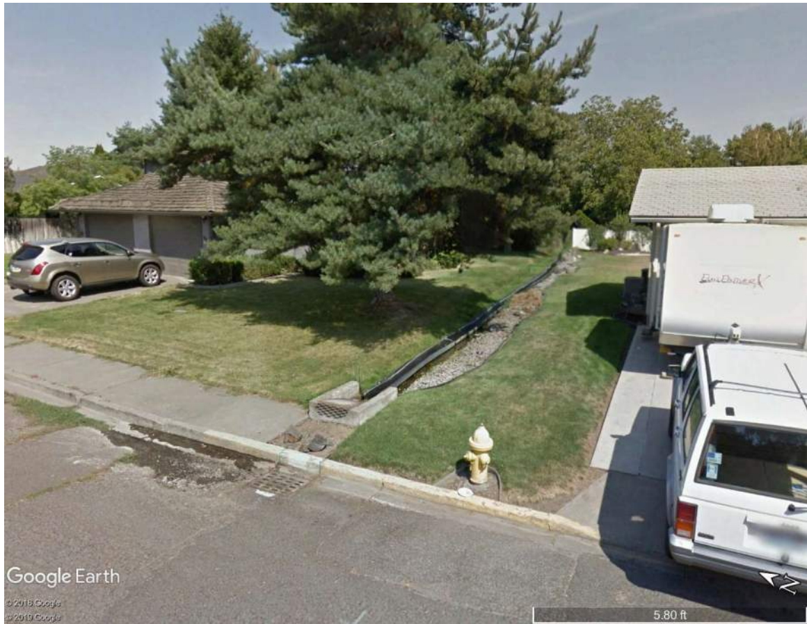
Photograph 4-5. Outfall #55 - Cedar Avenue Catch Basin (Google Earth)
