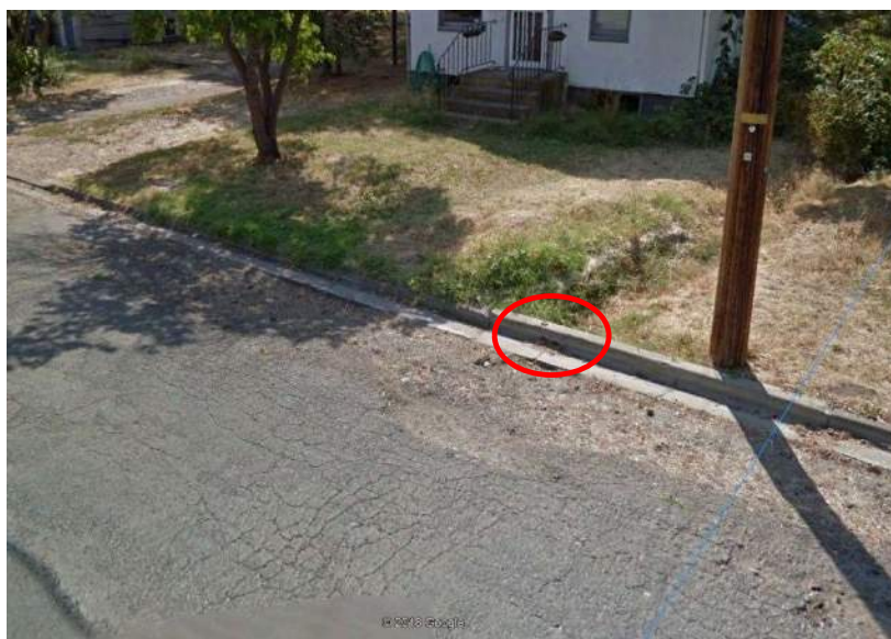
Photograph 3-4. Outfall #88 – Core-drilled curb (Google Earth)
