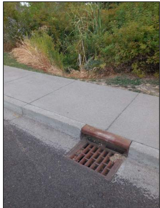
Photograph 2-19. Outfall #1 - Catch Basin Inlet - Looking west
