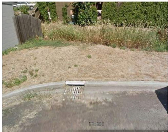
Photograph 1-7. Catch Basin ID#3
