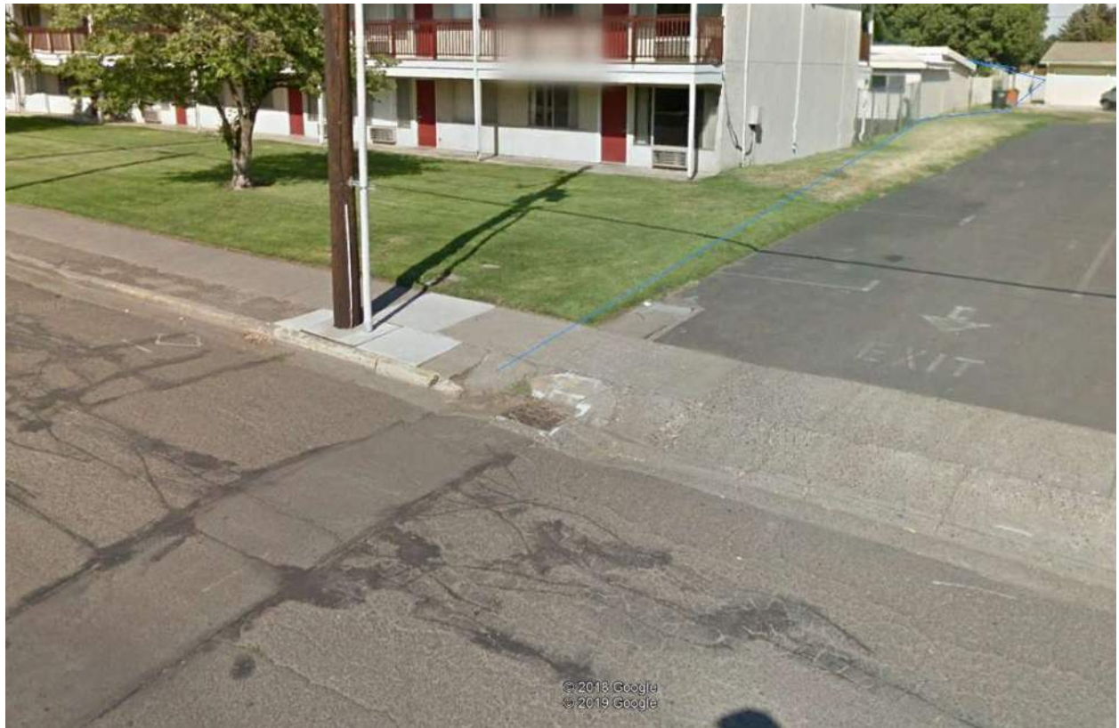
Photograph 4-9. Outfall STRUCT 237 N College Avenue (Google Earth)
