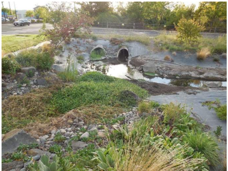
Photograph 2-7. Stone Creek Culverts beneath Meadowbrook Street - Outfall to West (far side)
