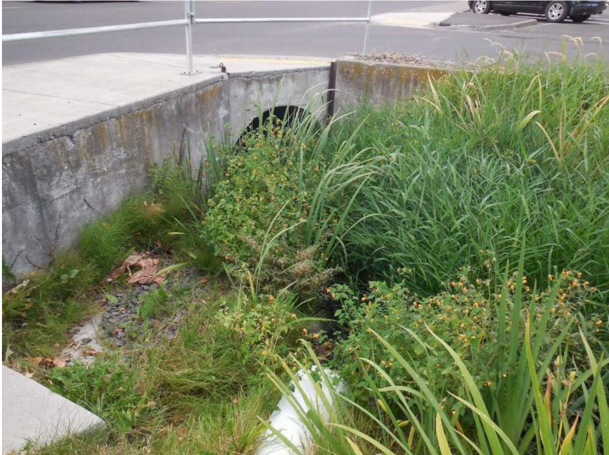
Photograph 1-14. Outfall 79, 85, 86, 87 - Looking West - Larch Avenue
